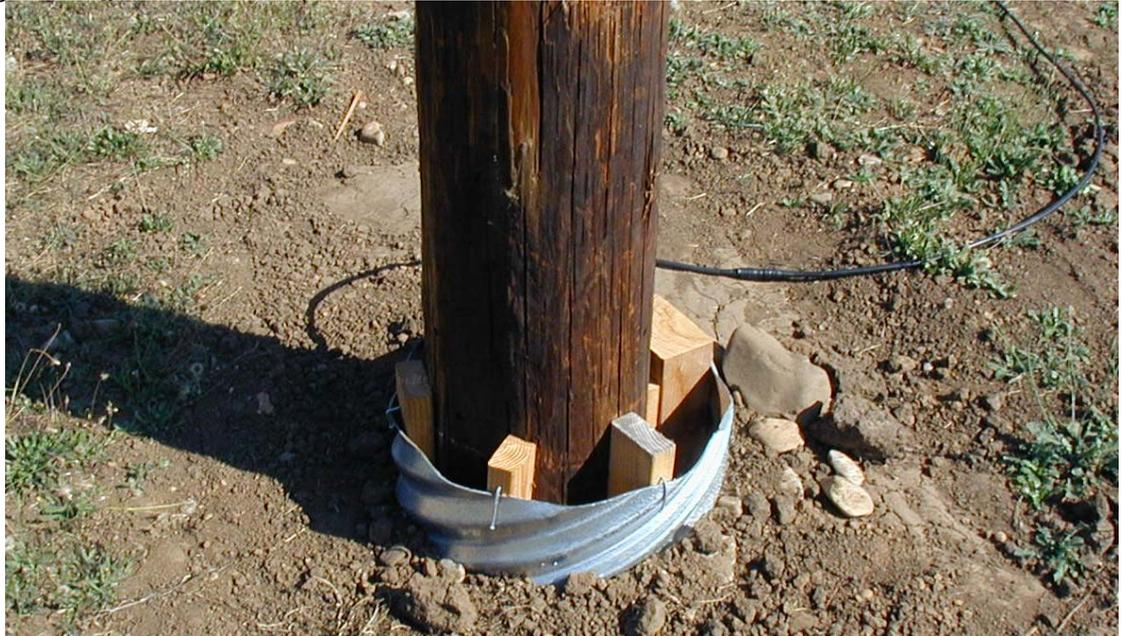
The bottom of the pole is inserted into a section of 18" diameter, 7' long corrugated steel culvert as shown above. The culvert is buried in the ground as shown above.
