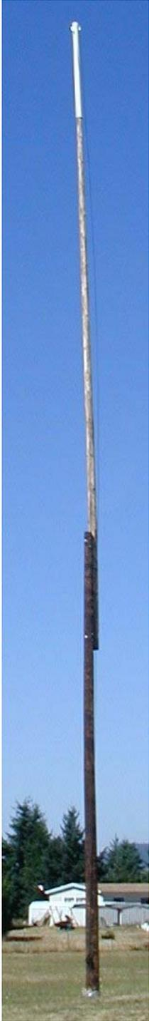
On the left is a picture of a typical pole assembly. On the bottom there's a 50' treated utility pole. Bolted to the top of the utility pole is a smaller diameter 40-50' untreated pole with 10' of 6" PVC pipe covering the top. The pipe serves several functions: it makes the pole taller, it shelters the top of the pole from the weather (the part of the pole inside the pipe is treated) and it puts an insulator at a point which is often at very high voltage in a short top-loaded vertical.
