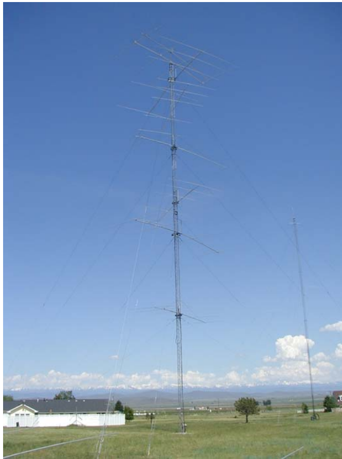
Figure 4, towers 3 and 4, looking a bit north of east.
